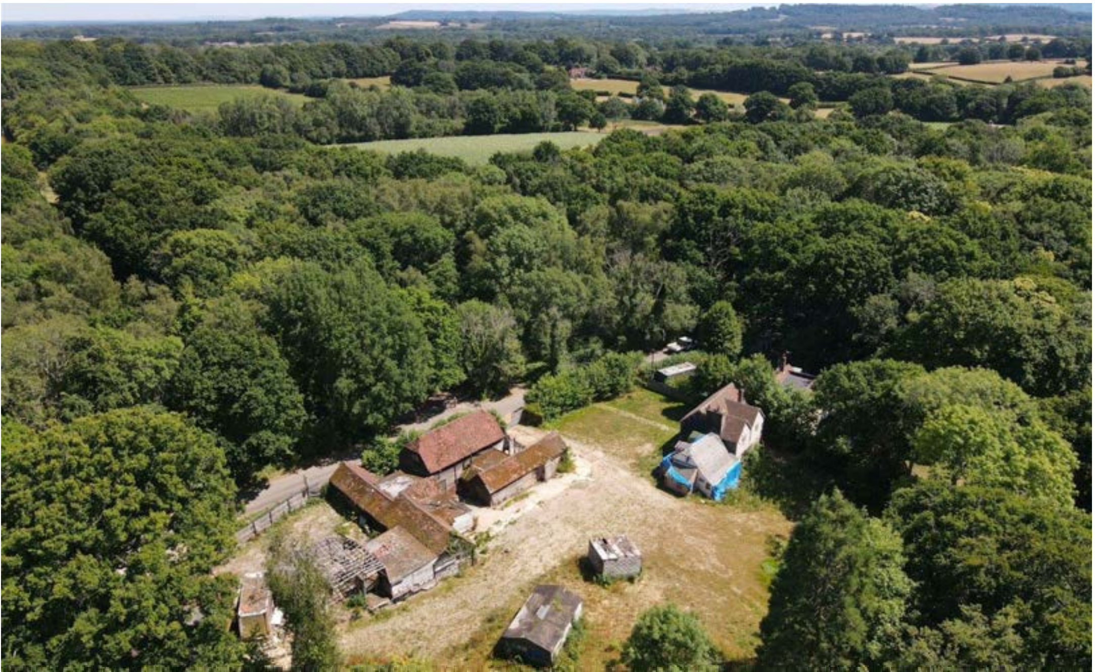
Windfall Wood House and Tappers Barn, Lurgashall GU28 9HA Freehold
