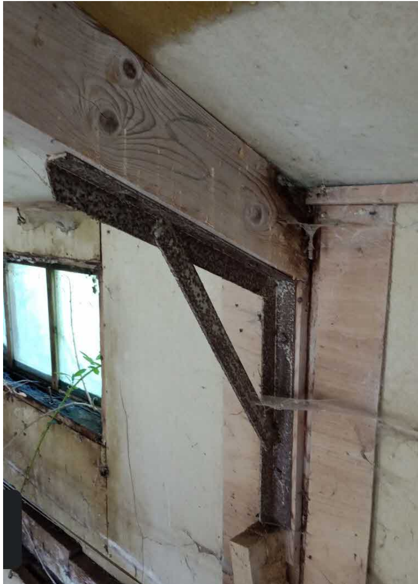
Steelwork truss eaves connection detail
