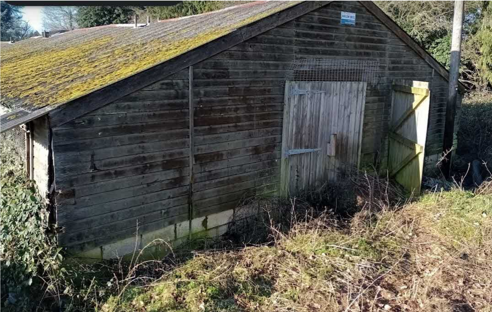
External blockwork lower walls and timebr clad timber external walls and metal sheeting roof (Rear wall)
