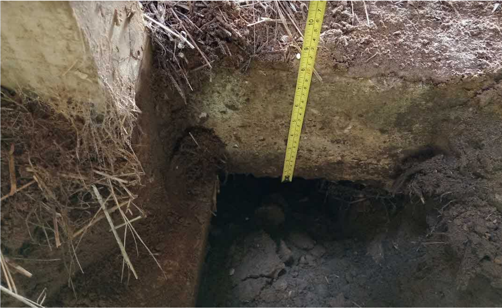
Concrete ground floor slab revealed in hole, 200mm thk
