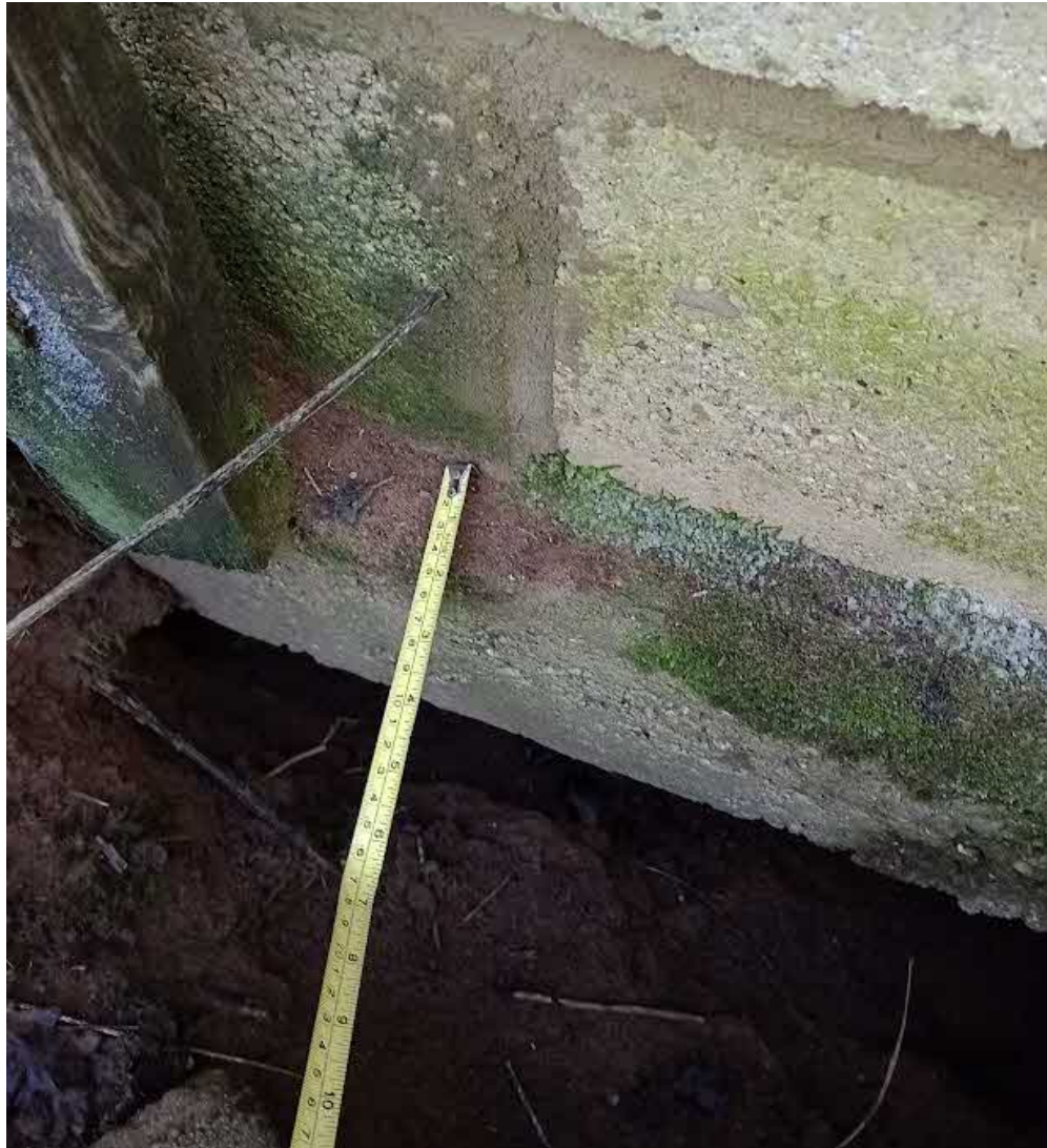
Concrete foundations revealed in hole on site, 200mm thk concrete
