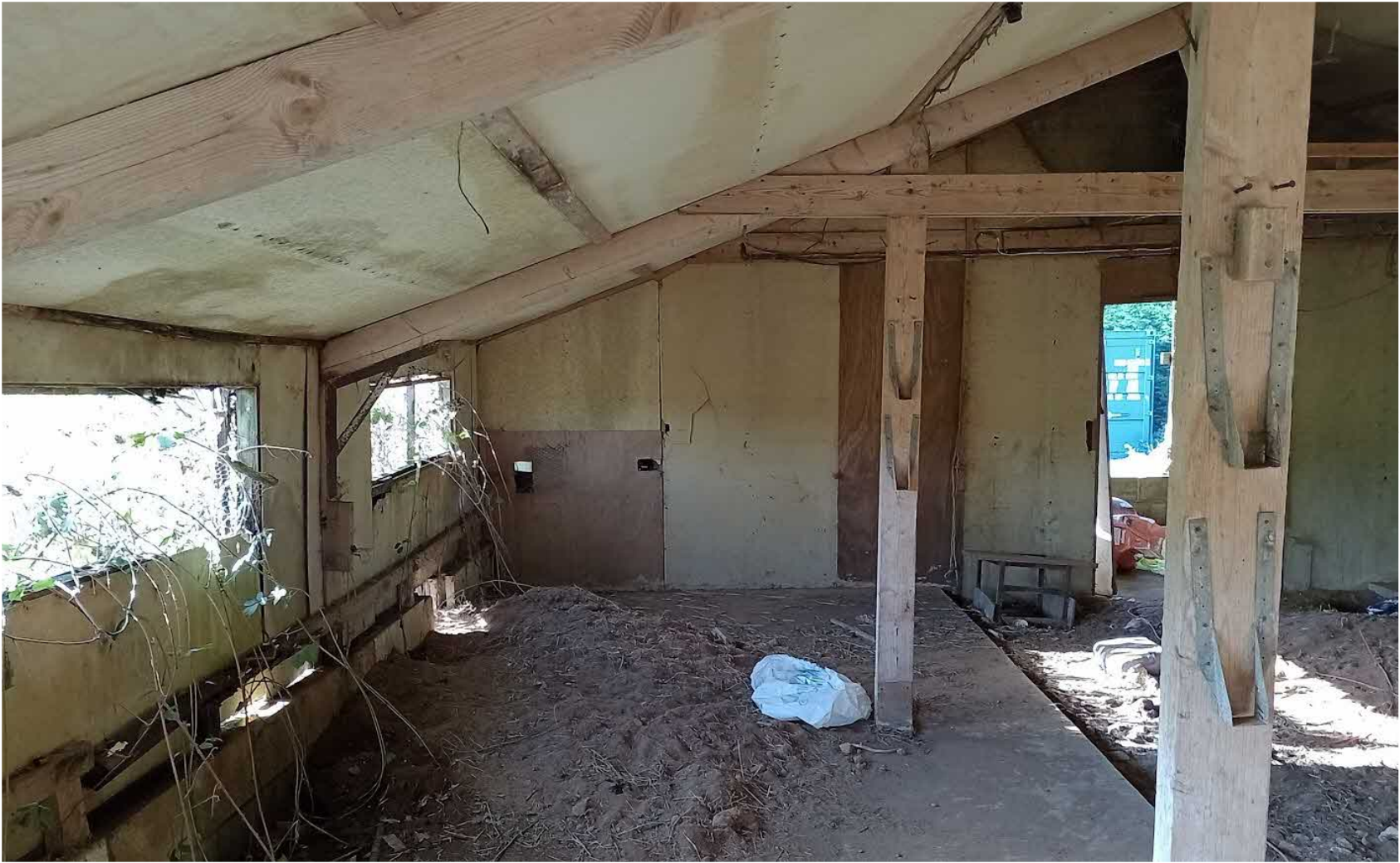
Timber roof trusses and posts supported on slabs
