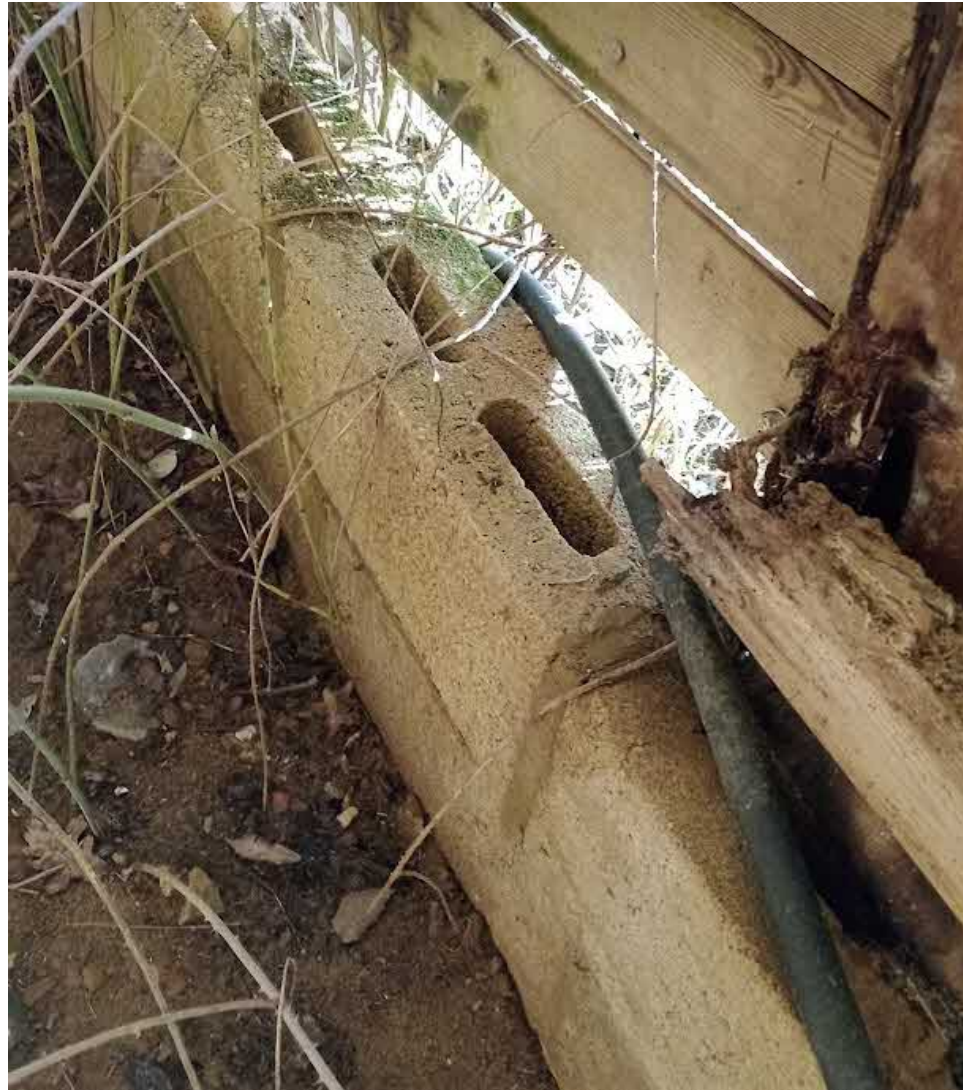
External lower hollow blockwork wall (140mm thk)
