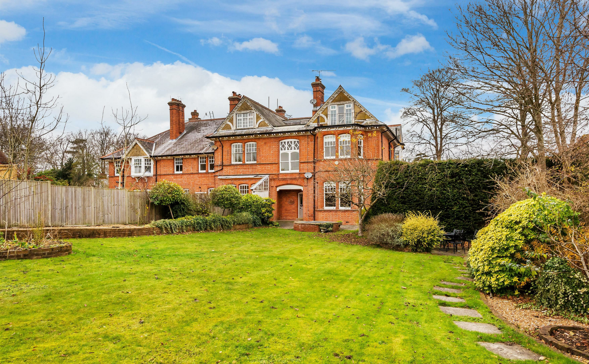
Firfield Lodge, Grove Road, Guildford, Surrey
